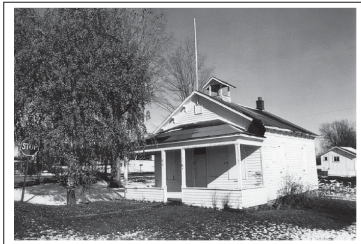
Q-40: Ballou Schoolhouse Ouderkirk Road & Tryon Road Date of photo: Nov., 1993 View: looking NE
