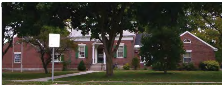
Ainsworth Memorial Library on South Main Street in the Village of Sandy Creek.
