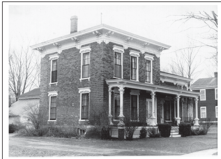
Q-62: Mark V. Sellis House 9278 North Main St., Sandy Creek Date of photo: 1976 View: looking SE Photo by: Marie Parsons
