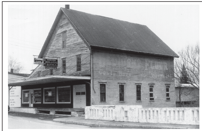
Q-78: Sancona Builders Supply Co. North Main Street, Sandy Creek Date of photo: 1976 View: looking SW Photo by: Marie Parsons
